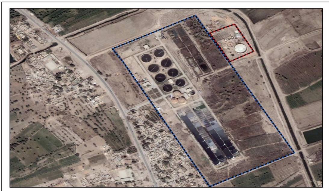
Figure (1): Al-Barakiya Treatment Plant in Najaf Governorate.
